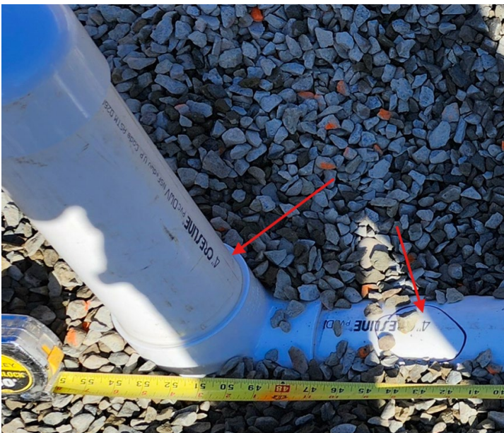
Example of main drain piping manifold.
